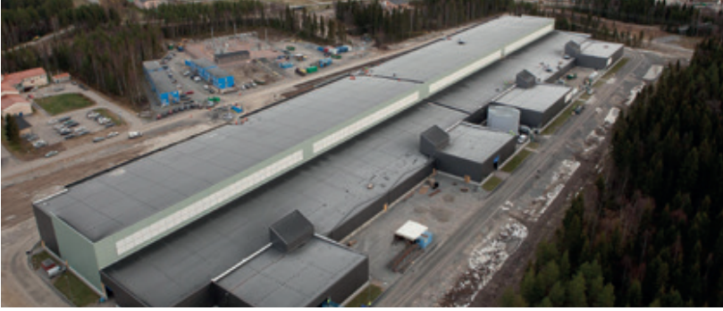
Data centre building
